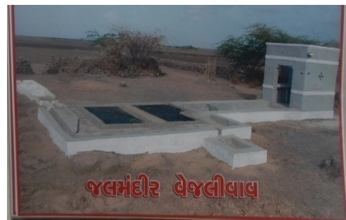
RESTORATION WORK OF STEP WELLS
