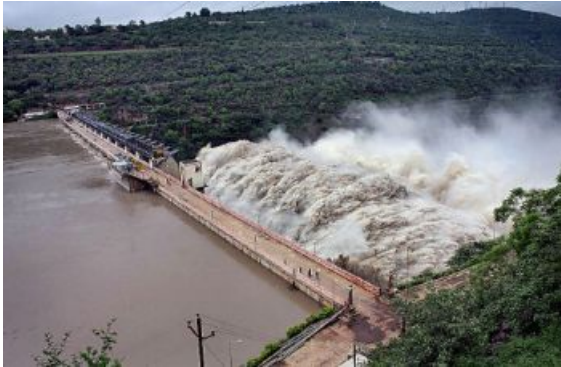
OVERFLOWING SRISAILAM DAM IN OCT -2009 FLOODING
