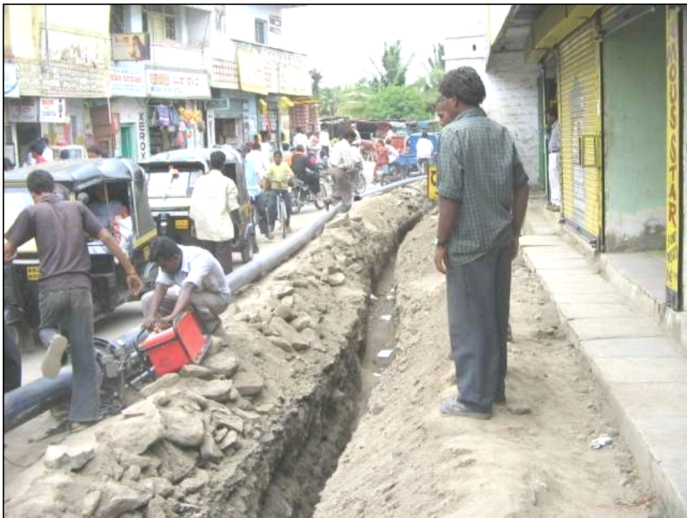
Figure 4. Easy and fast installation of PE pipes in crowded area. Joining carried out outside the trench requires lesser trench width, saves trenching cost.
