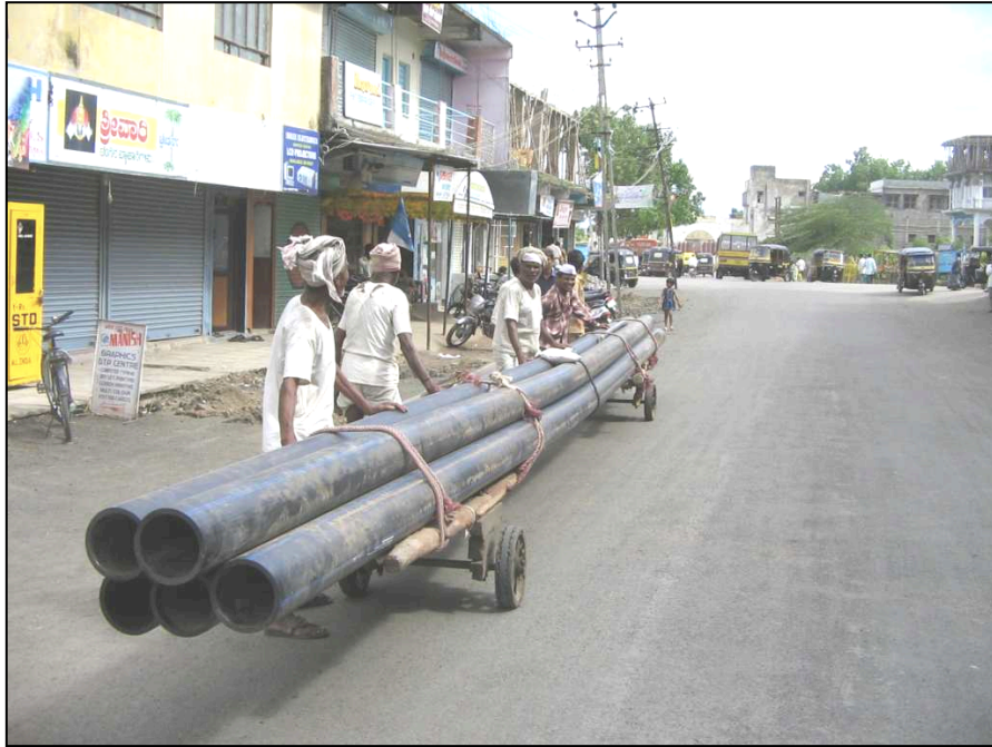
Figure 3. No heavy lifting equipments needed for secondary site transportation of PE pipes.
