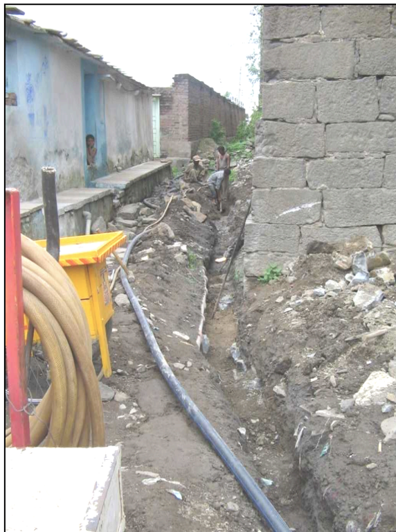
Figure 6. PE pipes are available in coil up to 1km length, results in lesser joints and faster installation in congested area.
