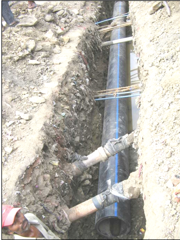
Figure 5. Inherent flexibility of PE pipes simplifies installation without disturbing existing utilities.
