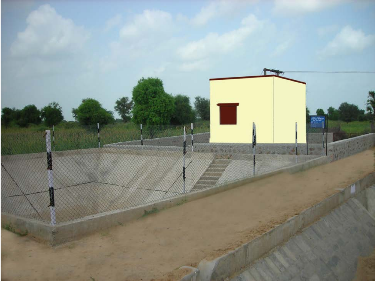
STILLING BASIN( DIGGI) AND PUMP HOUSE
