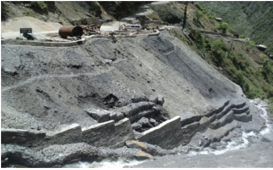
Figure 1. Stepwise phases of restoration of Muck dumping
