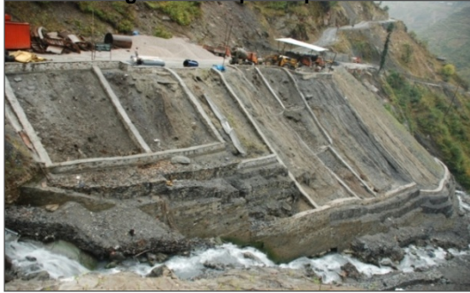
Figure 1. Stepwise phases of restoration of Muck dumping
