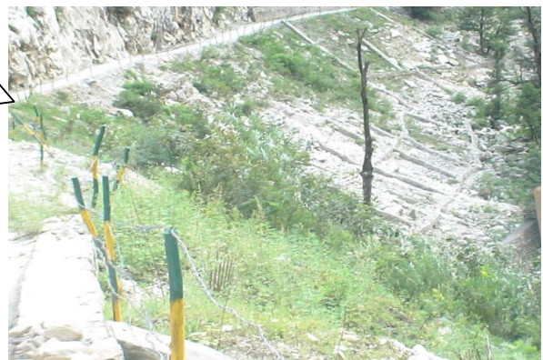
Figure 3. Restoration measure at Muck dumping site-5 and additional muck dumping site-5
