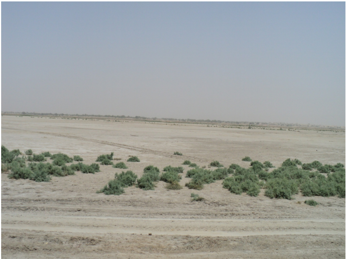
Photograph 2. Water Logged area of Rajasthan Feeder
