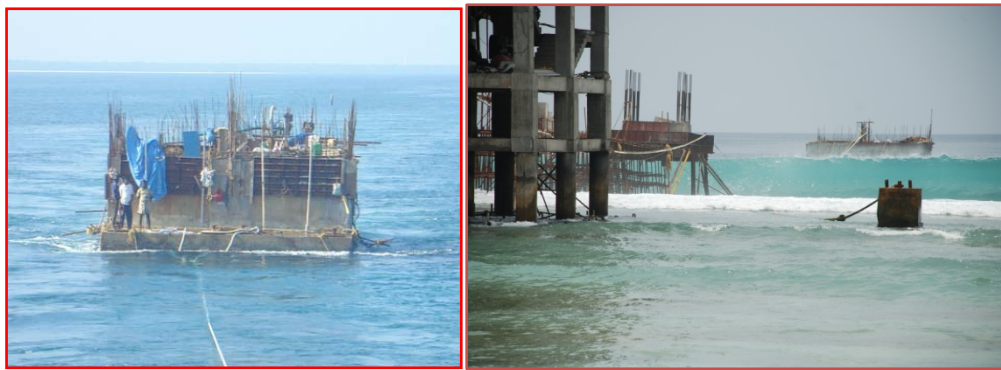
Fig. 3 Views of Sump during its Tow (left) and Wave activity in the Breaker Area (right)
