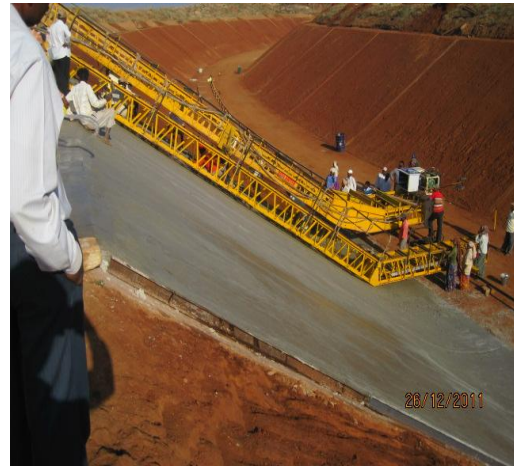
Fig 7: CC lining in canal (Km 20)
