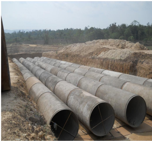
Fig 6: Raising main near Muttenkoppa ( NR Pura Tq.)
