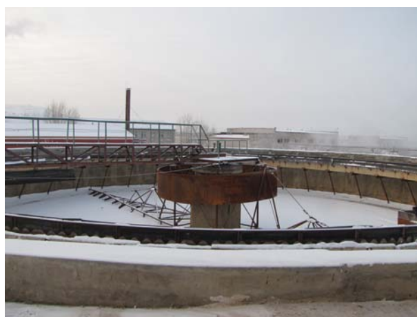
Figure 7: State of Darkhan's central WWTP
