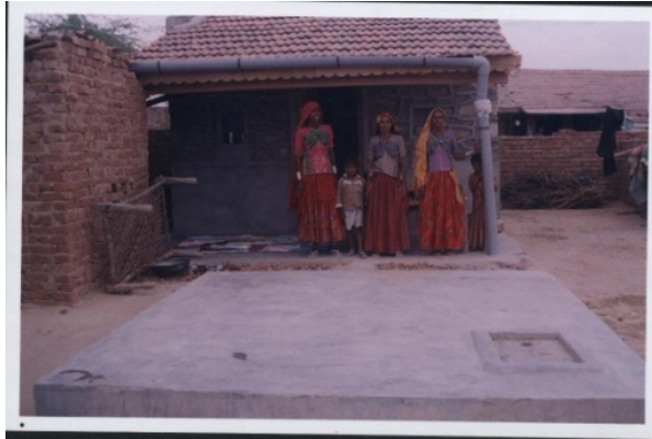
Figure 10. Roof Rain Water Harvesting Tank
