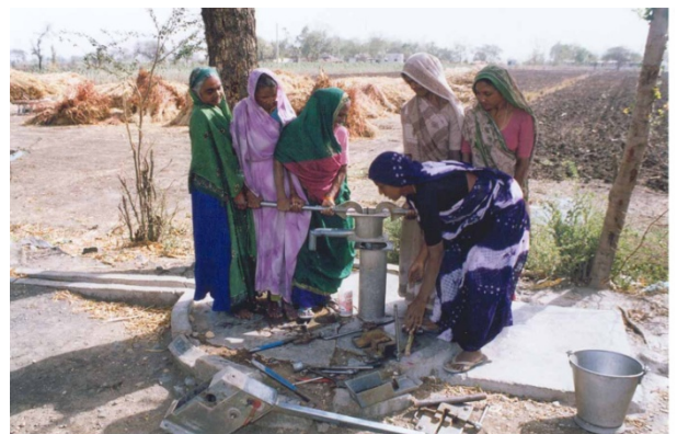
Figure - 5 Hand pump Repairing work
