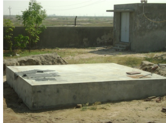
Figure 10. Roof Rain Water Harvesting Tank
