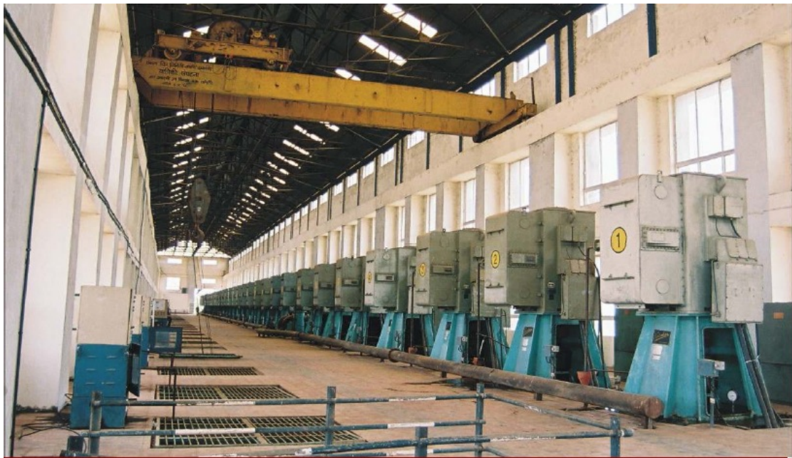
Figure 8: Photograph of completed Mhaisai Pumphouse
