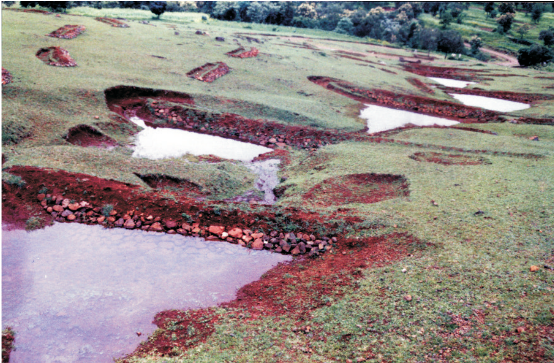
(Gully Plugging Structures - 834 Nos.)
