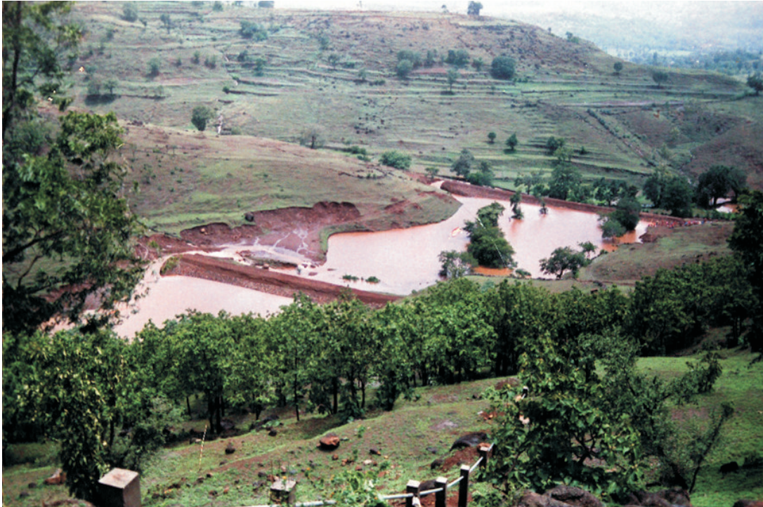
(Water Harvesting Structures - 20 Nos.)
