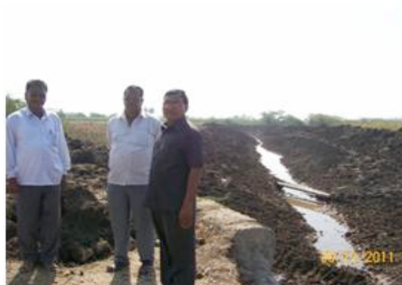
Figure 10C: Main Drain After Work
