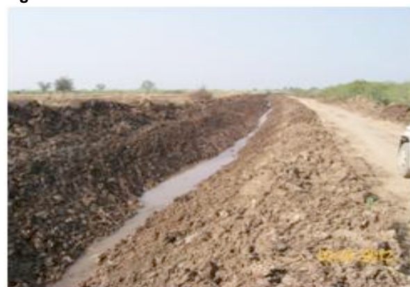
Figure-10B : Drainage Scheme Functioning After work.
