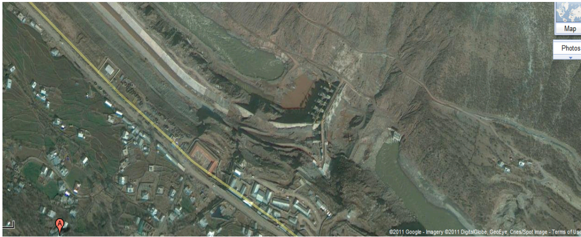
FIG 1: SATTELITE PICTURE OF URI II HYDRO-ELECTRIC PROJECT, DAM SITE, UNDER CONSTRUCTION, IN THE MOUNTAINS OF VILLAGE URI, BARAMULLA.
