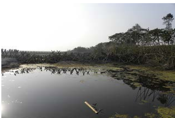
Fig.-4: Siltation induced due to RCC porcupines
