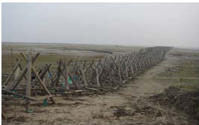
Fig.-3: Reclamation of land due to porcupine screens
