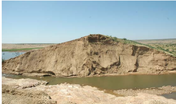
Fig 1: Homogeneous embankment section
