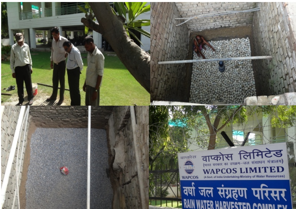
Photograph showing Injection Well and Laying of Filter Material
