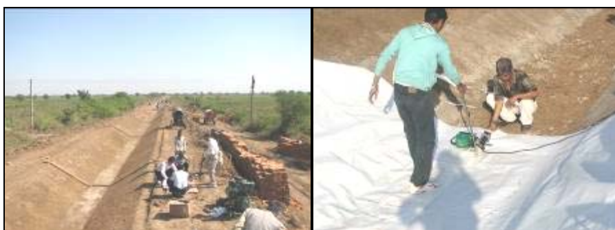
Photos – 5 and 6 Preparation of Canal Section and Heat Sealing of Geomembrane
