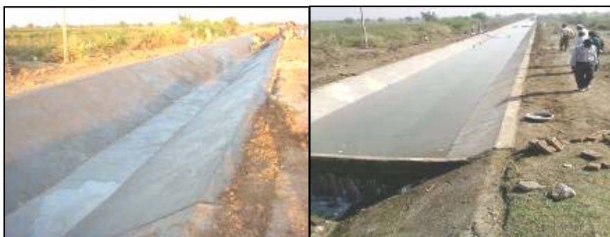
Photos – 7 and 8 Completed Canal Section
